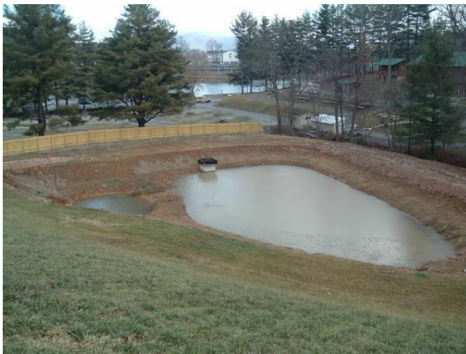
Figure 3. 12 Detention pond (Stormwater Management)
